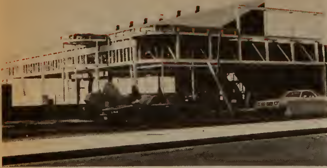
Massachusetts Avenue Station superstructure under construction.
